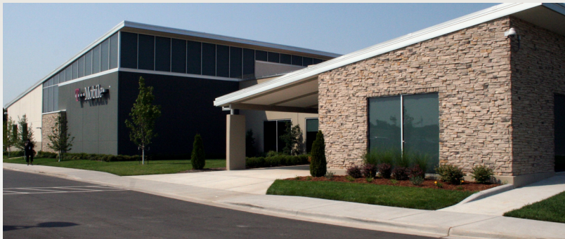
T-Mobile USA opened their 800 employee center in 2006 and now handle more customer service calls than any other T-Mobile facility.
